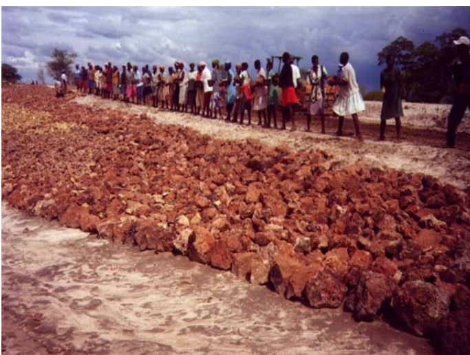
Dongamuzi (Nhangano dam) stone pitching
